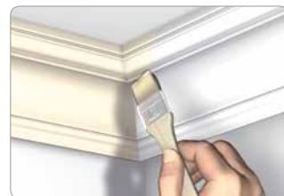
Paint the cornice in the same color as the wall and/or ceiling
