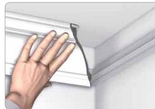
Attach the cornice to the rail and the ceiling
