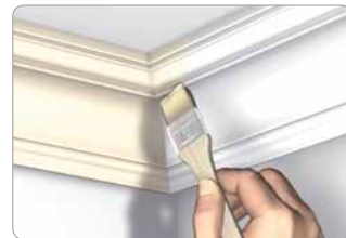
Paint the cornice in the same color as the wall and/or ceiling
